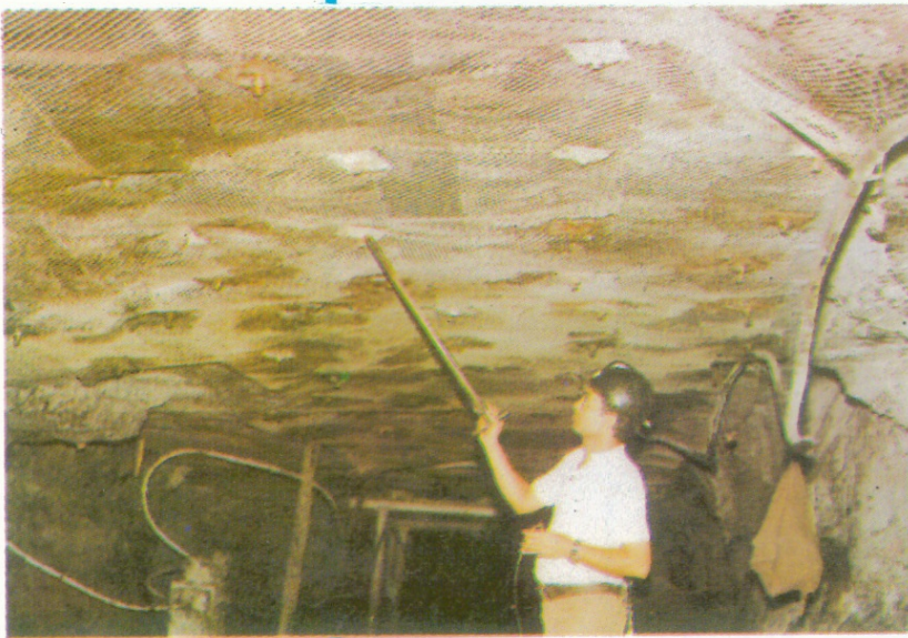
Combination of wire netting and Roof bolting
