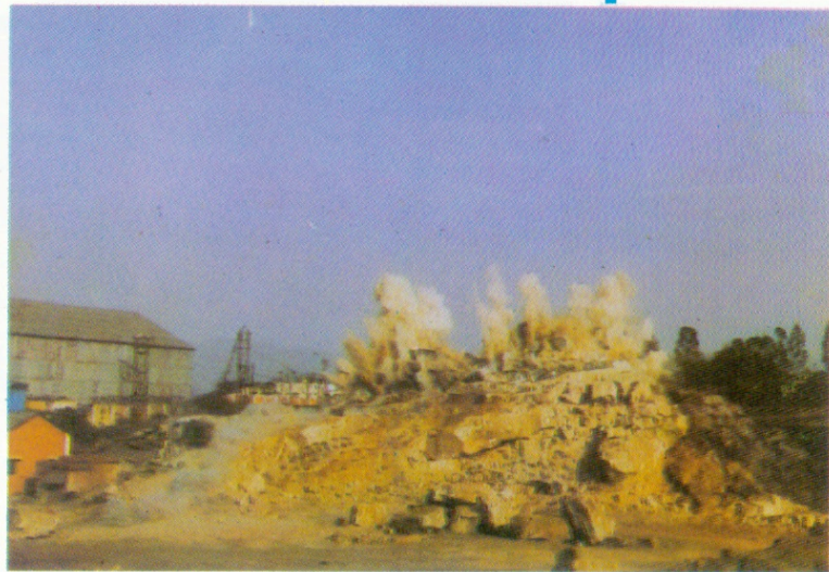
Surface blasting near built-up structures
