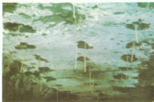
Cable bolted roof before blasting of the roof coal
