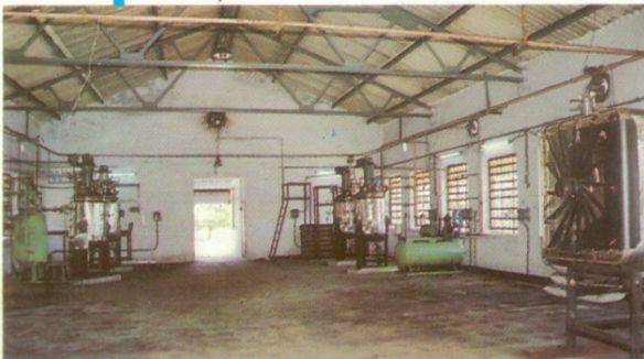
A full view of installed Biofertilizer Plant (100 T/Annum)
