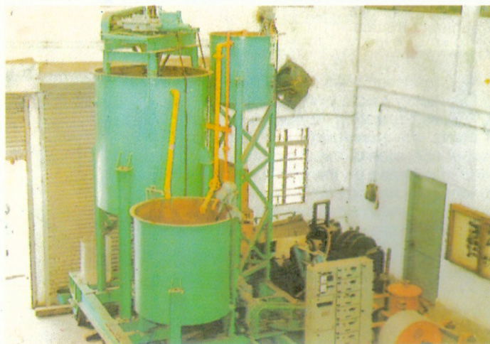
Pilot Plant showing high rate thickener — continuous working system
