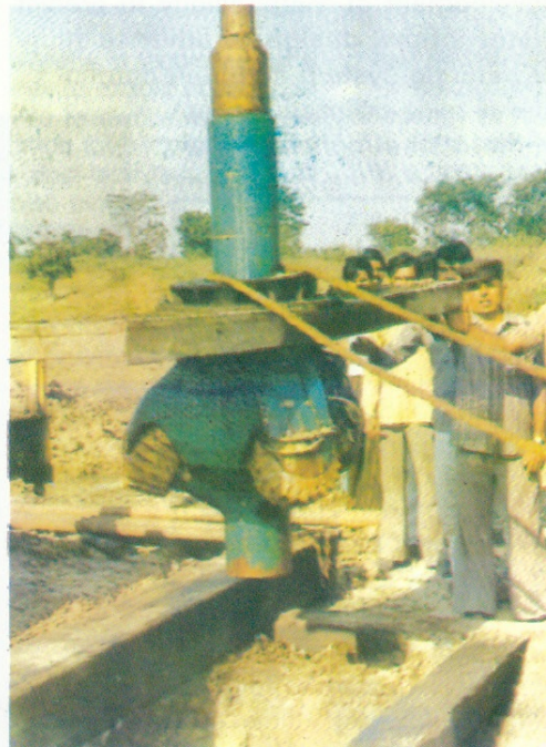
36" dia hole being drilled at Mahabir colliery for rescue operation
