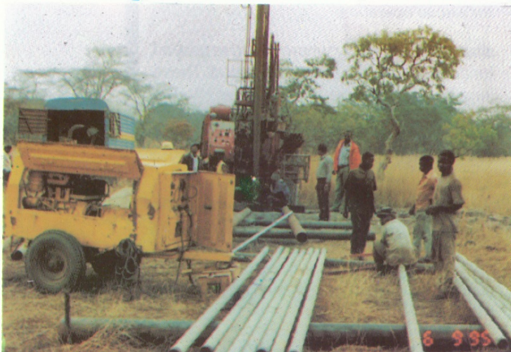
Well construction at Mchuchuma Project, Tanzania
