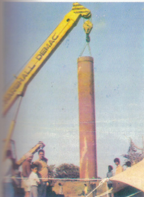
Large dia casing being lowered at Mahabir colliery
