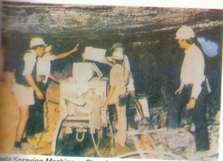
Seela Spraying Machine — Charging of Sealant
