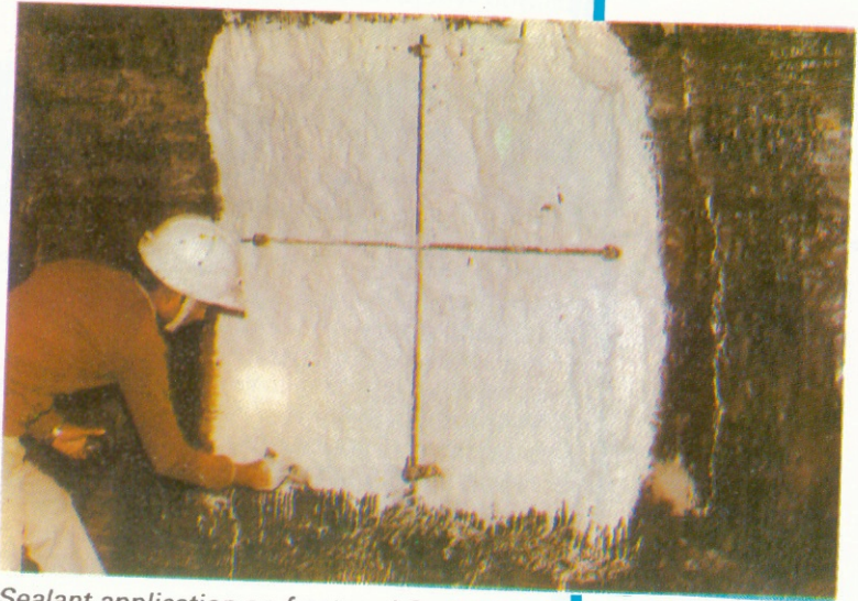
Sealant application on fractured Coal Pillar
